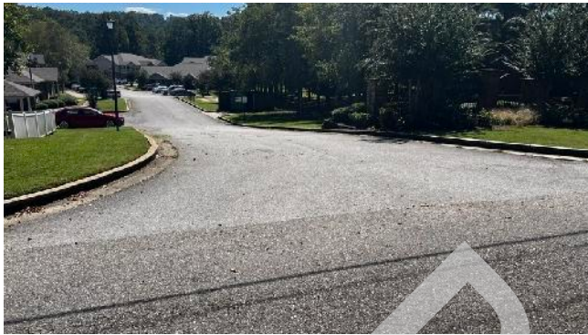
Subject Property entrance
