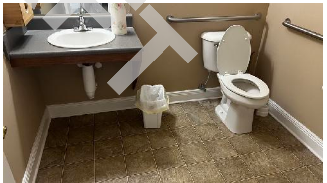
Leasing office restroom
