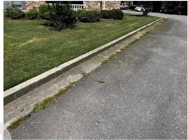
Asphalt paving and concrete curb
