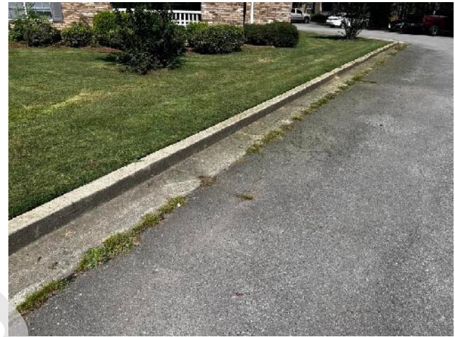
Asphalt paving and concrete curb
