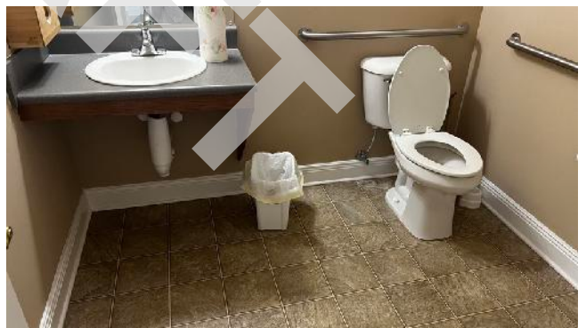
Leasing office restroom
